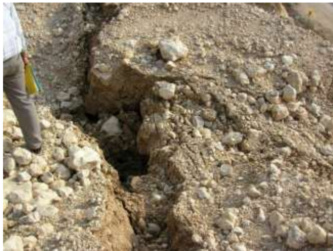
Figure 3.31 Cracks on top the slide mass confirming changes of further movement
