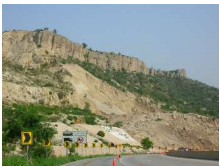
Figure 3.25 A view of potential land slide site along the alignment
