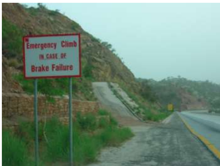
Figure 3.17 Emergency Climb Lane for safety
