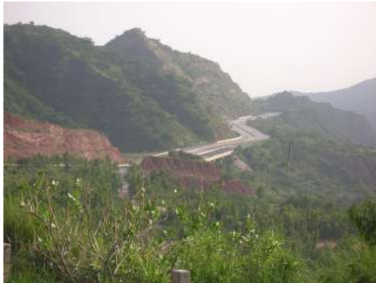
Figure 4.2 View from Km 229 of negative slope at Km 227
