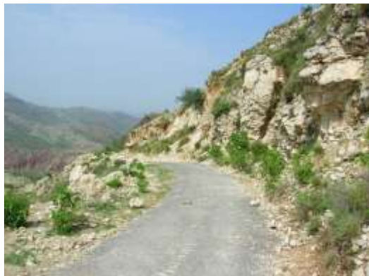
Figure 2.8: View showing steep gradients on Route R-1
