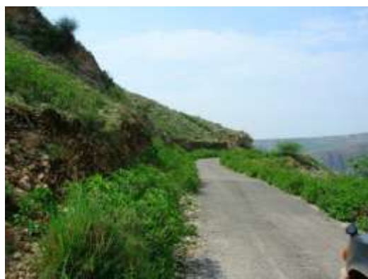
Figure 2.11: View showing steep gradients on Route R-1
