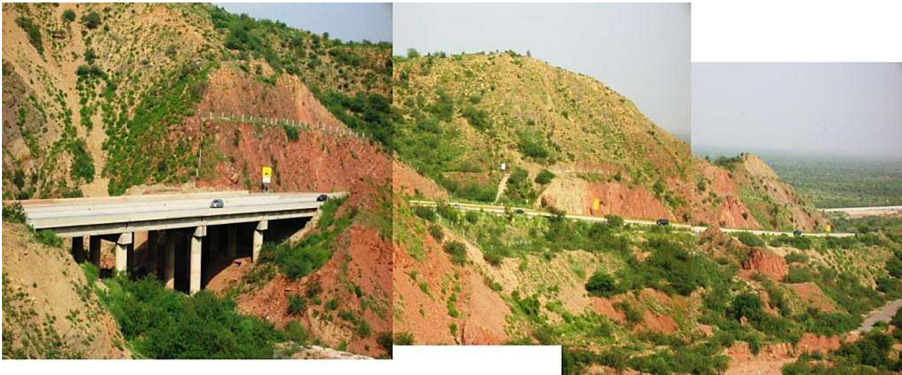
Figure 4.1 A panoramic view of first steep rise of nearly 7% at start of Salt range (Lahore end) leading to Bridge BD-12C3
