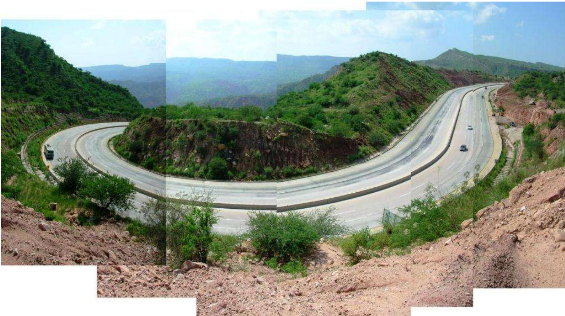
Figure 4.4 A panoramic view of double hairpin bend with 7% vertical slope at km 229 creating a black-spot
