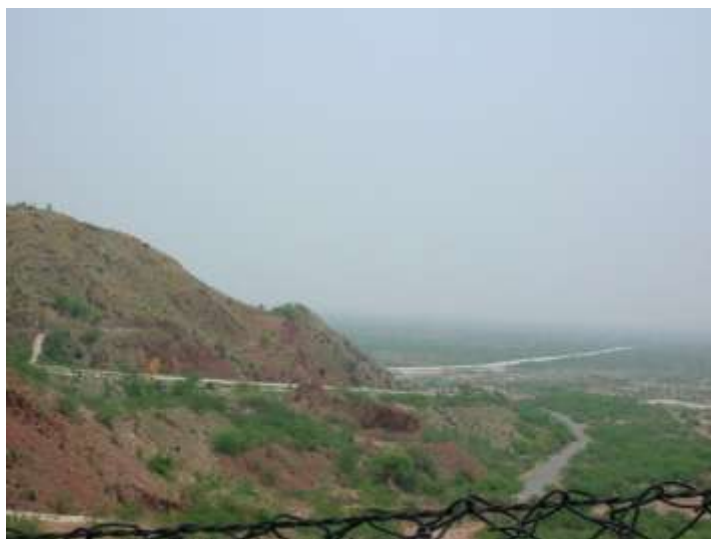
Figure 3.10 Side view of the motorway showing severity of the slopes
