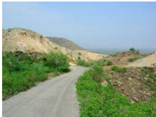
Figure 2.9: View showing variable geology & cut up terrain on Route R-1
