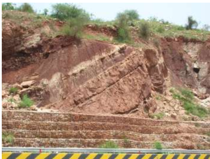
Figure 3.23 RCC wall to prevent falling rock pieces from affecting traffic safety
