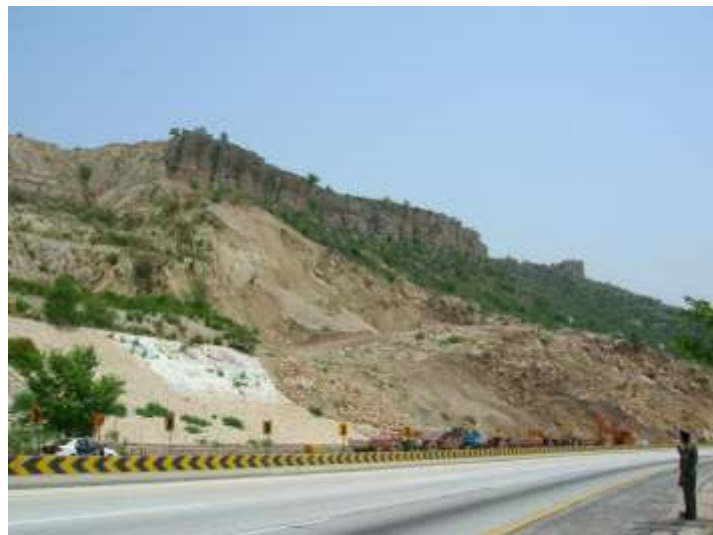
Figure 3.27 Work in progress to keep southbound carriageway open to traffic
