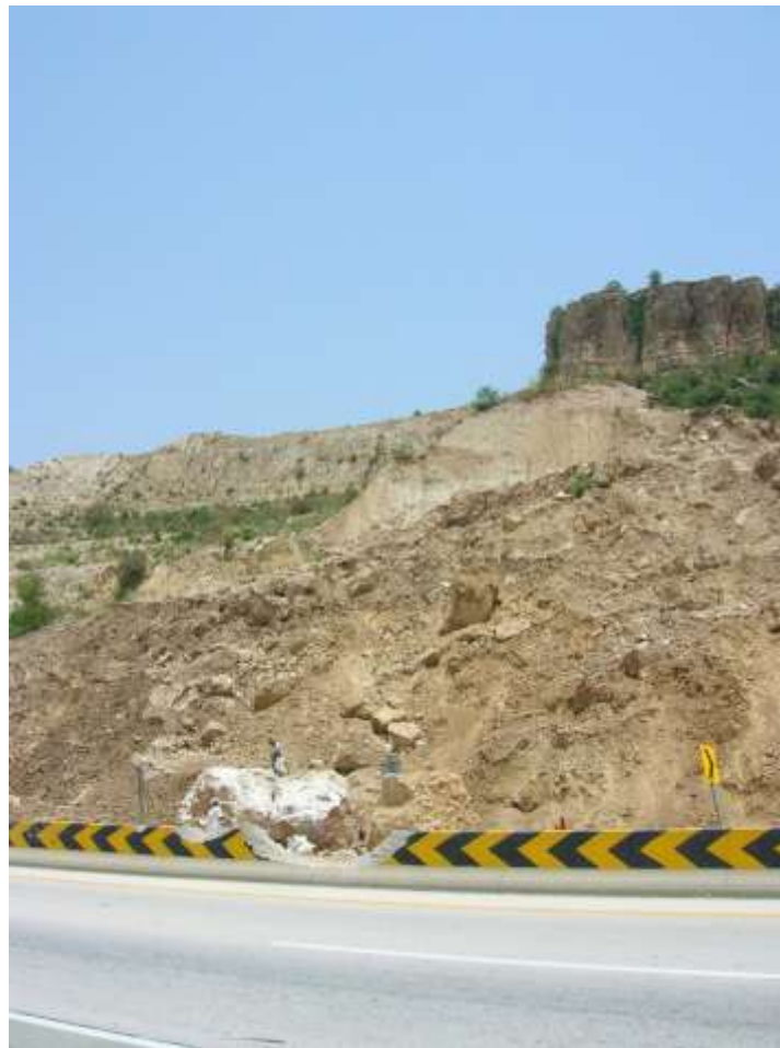
Figure 3.28 Severe Damage caused to central NJ Barrier by falling boulders
