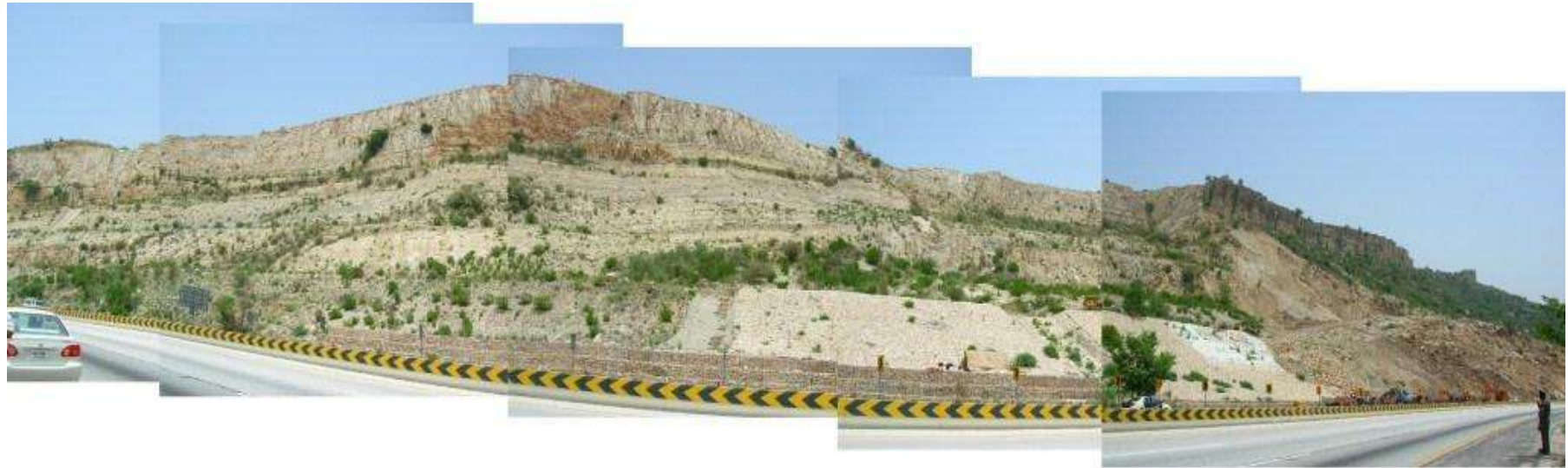
Figure 3.34 Panoramic view of the Heavy Cut at Simbal showing high Cliffs, rock benching & protection works. Land slide is visible in extreme RHS end
