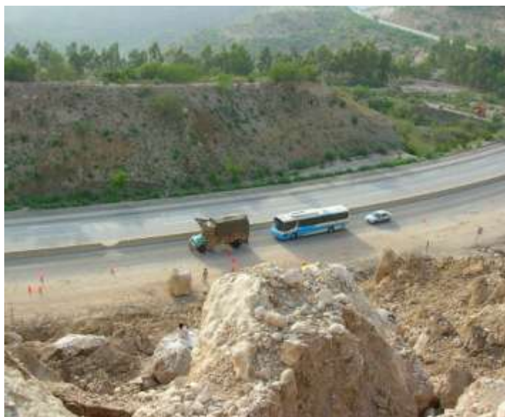
Figure 3.19 Vehicular traffic exposed to landslides and rock falls
