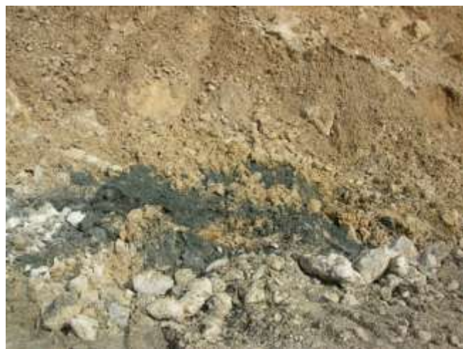
Figure 3.29 Blackish / Greyish liquid seeping at bottom of the land slide area
