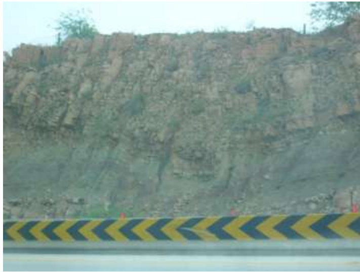
Figure 3.22 A view of rock fall area along the alignment
