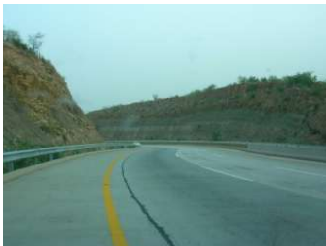
Figure 3.14 Combination of vertical slope & sharp "s" curve
