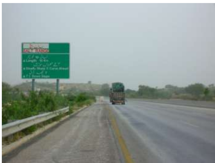
Figure 3.4 Sign Board heralding speed restrictions on south bound traffic
