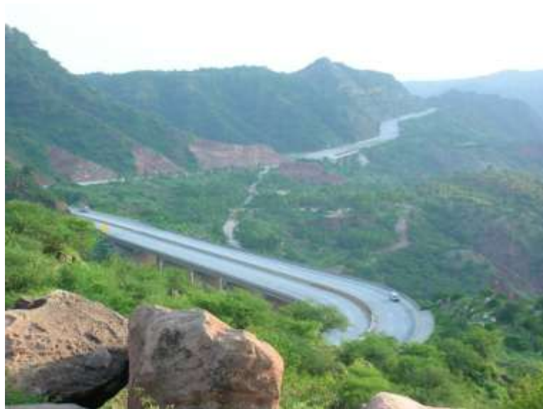
Figure 4.3 View showing negative slope at Km 227 followed by steep 7% slope leading to Bridge BD-12C6 at Km 229
