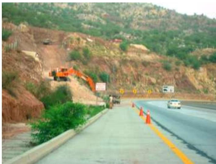
Figure 3.16 Emergency Climb lane being improved
