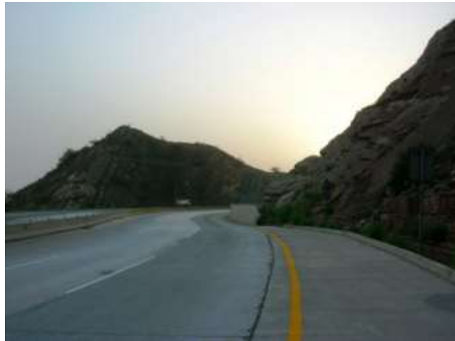
Figure 3.7 The combination of steep slope & sharp curves
