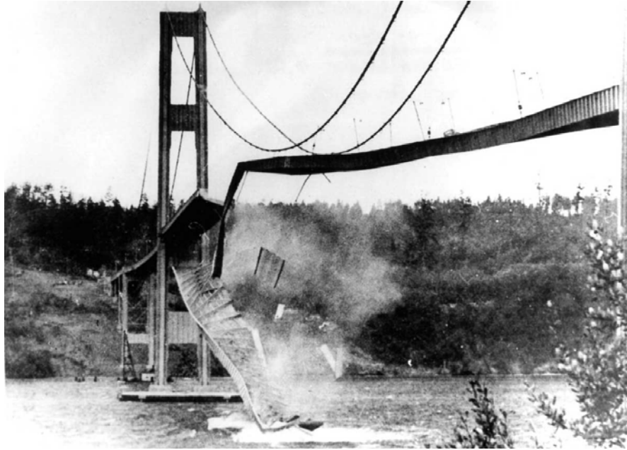
a) Tacoma Narrows Bridge collapse due to resonance [12]
