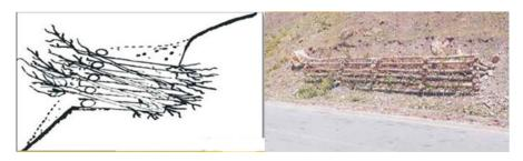
Fig. 8.4 Vegetated timber crib wall
