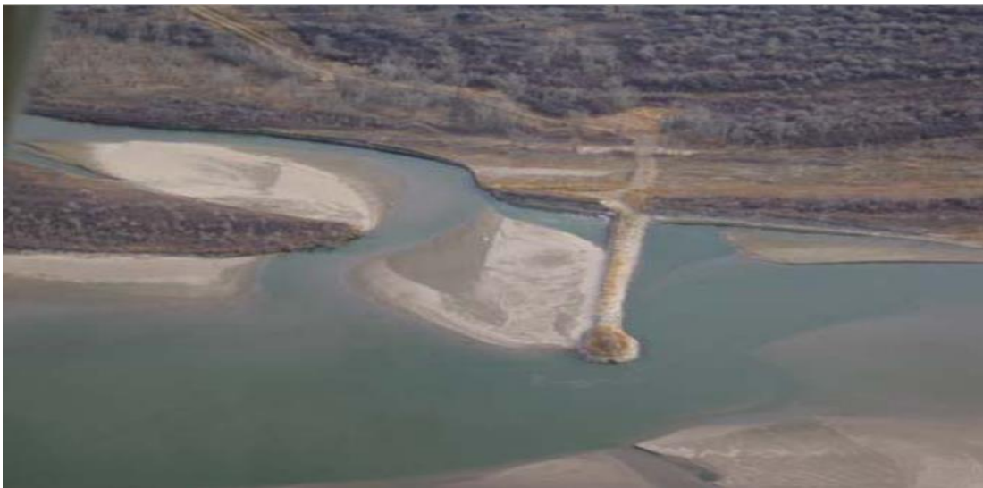
Figure 1.1: Single spur on the Saskatchewan River in the vicinity of the pike lake water intake
