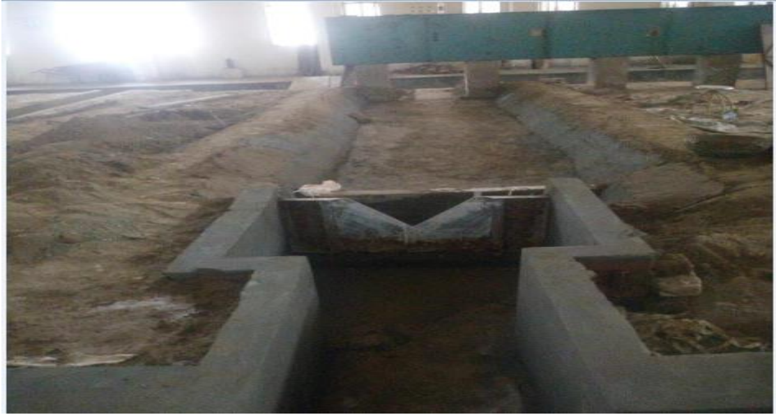
Figure 3.1: Experimental channel constructed in MT- Hall
