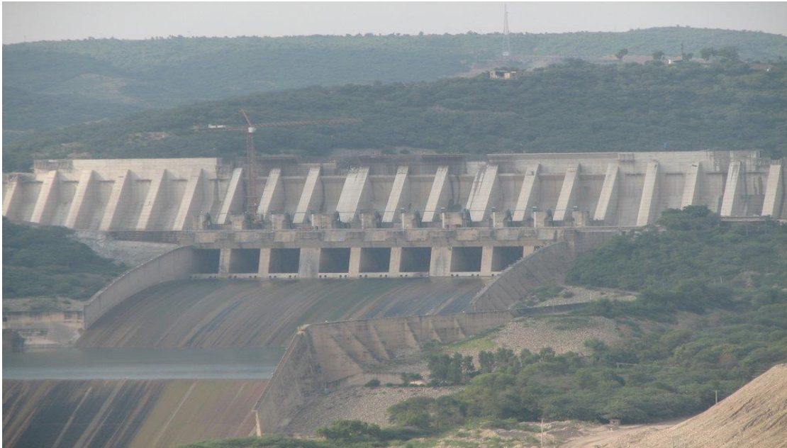
Figure 2.1 Spillway of Mangla dam
