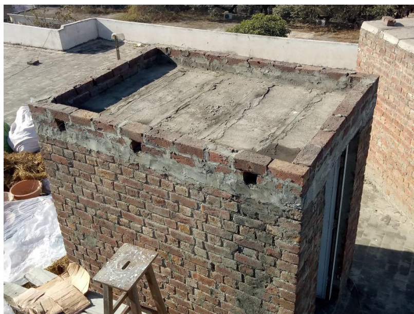
Fig-2. 11 Cleaning of 8 inch BCP roof
