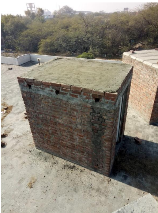
Fig-2. 22 PCC placement on 8 inch BCP roof
