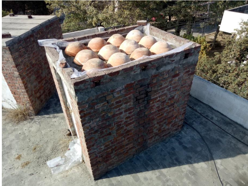
Fig-2. 19 Placement of 6 inch Burnt Inverted Clay Pots on roof
