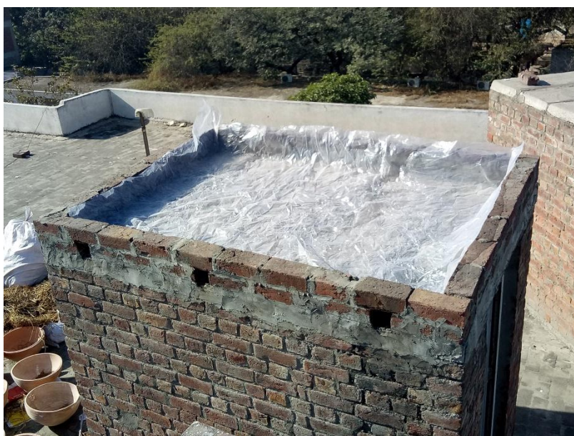
Fig-2. 13 Water proofing sheet on 8 inch BCP roof
