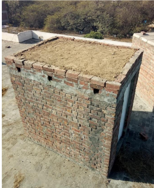
Fig-2. 20 Mud filling on 8 inch BCP roof
