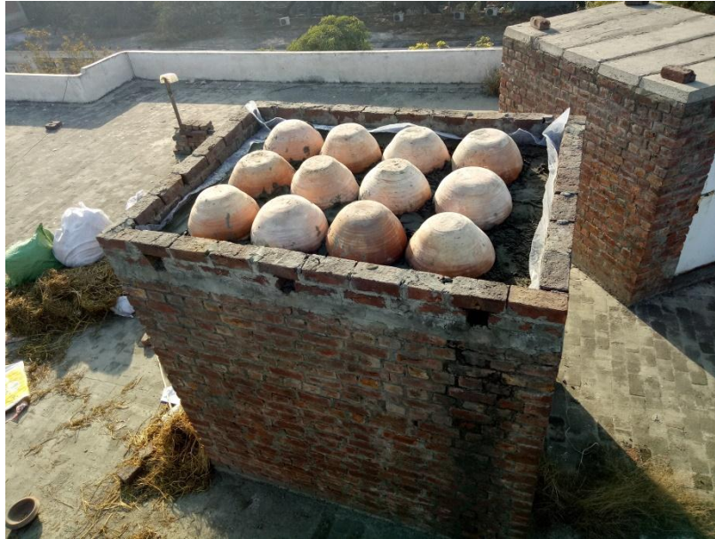
Fig-2. 18 Placement of 8 inch Burnt Inverted Clay Pots on roof
