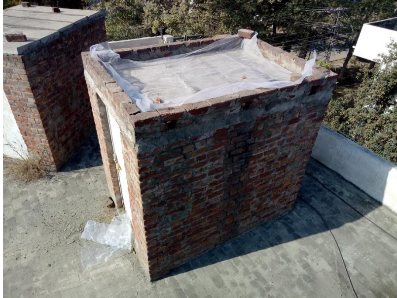
Fig-2. 14 Water proofing sheet on 6 inch BCP roof
