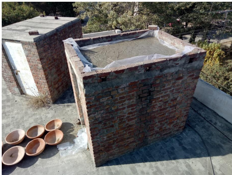
Fig-2. 16 Cement Sand (1:1) slurry on 6 inch BCP roof
