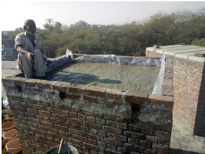
Fig-2. 15 Cement Sand (1:1) slurry on 8 inch BCP roof
