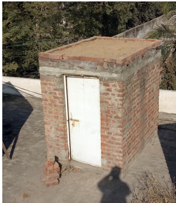
Fig-2. 21 Mud filling on 6 inch BCP roof
