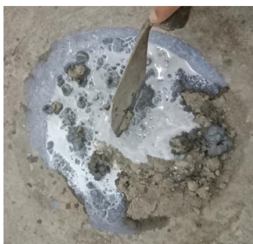
(d) Mixing of cement and SBR mixture
