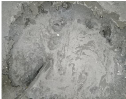
(c) Adding water to dry mix
